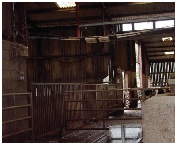
Figure 5: Antennae above passage way to the milking parlour.
