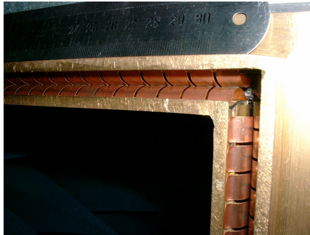
Figure 112 Appendix E: Example of a double row of spring fingers
